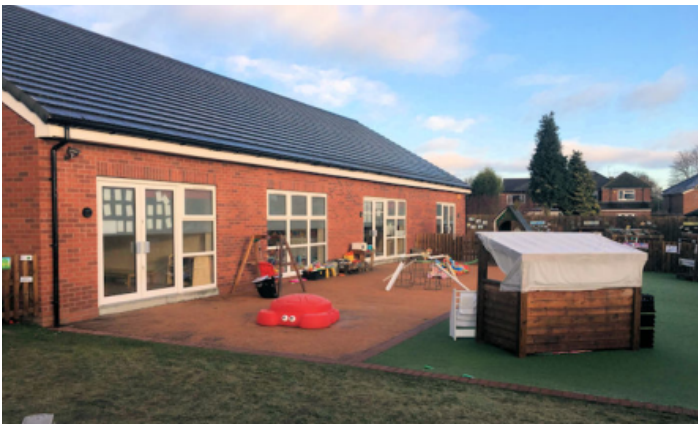
Above: Before the Canopy installation
