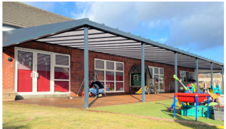
Above: After the Canopy installation
