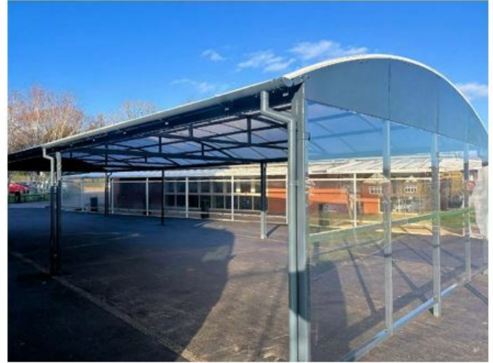
Above & Below: After the Canopy installation
