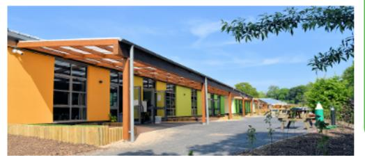
The canopy was further integrated with the building as it formed part of the rainwater management system of the building. The roof was designed to overhang the canopy so that the water drained off the main roof and into the gutter system on the canopy. This was done to simplify the system and will make maintenance easier by bringing the gutter height down – reducing both the short term and long-term costs of the building.
