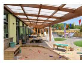
The canopy not only provides shelter from the rain, but the polycarbonate roof panels also offer shade and protection from the sun.
